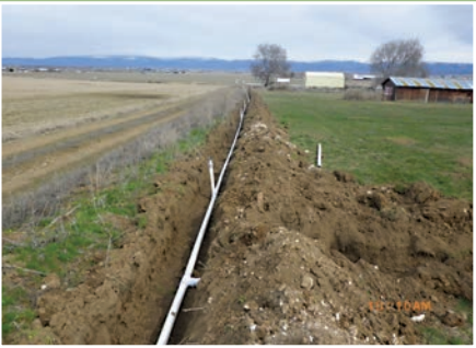
Below: Installing a mainline for a small sprinkler system
