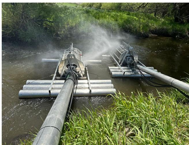
Figure 13. Fish screens installed on Cherry Creek for a pump diversion system. These are River screens, that do well in tributaries in the Kittitas Valley.
