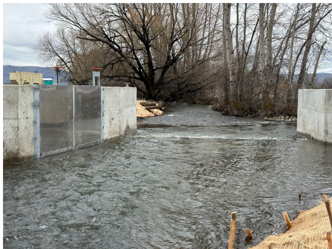
Figure 12. Fish screen (two silver panels on left side) installation on Coleman Creek to provide safe diversion of water for agricultural purposes and year-round fish passage.
