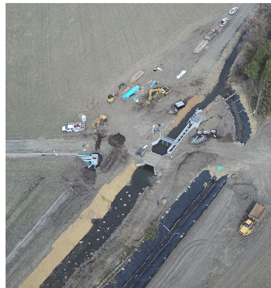
Figure 13. Fish screen and fishway structure construction at the upper diversion site (bridge) for consolidation of three diversions and correction of the fish barrier.
