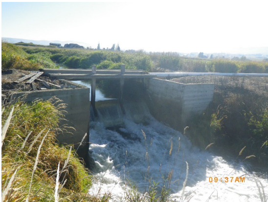
Figure 16. The lower irrigation diversion structure on Parke Creek before (left) and after (right) project construction. Removal of this barrier provided access to 2.3 stream miles of habitat.
