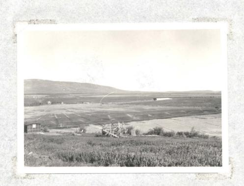
Rock drops were constructed in a gully which had been washed by excess waste water and spring run-off.
