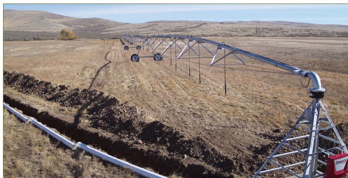
Most of the projects are installed in the fall and winter months. This is a center pivot sprinkler under construction. The mainline delivers water from the source to the pivot.
