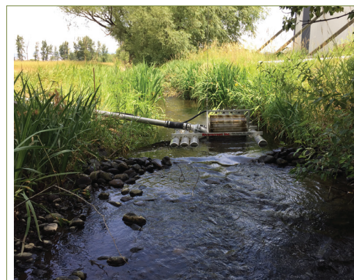
Fish screen (structure for water control) installed on an irrigation diversion serving a newly installed pivot system.
