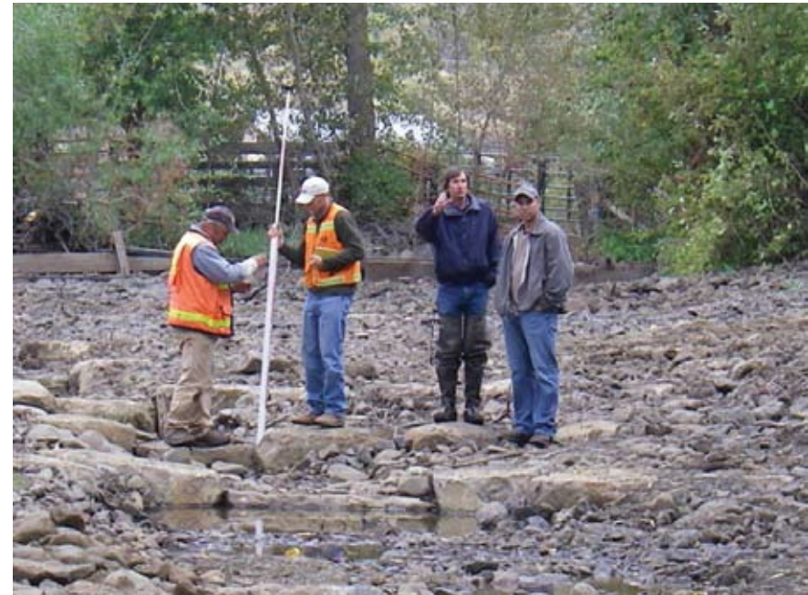
Don Shriner (KCCD), Mike Garello (HDR), Brent Renfrow (WDFW), and Brandon Drexler (Belsaas & Smith) check the elevations of the new installed rock weirs in Manastash Creek.
