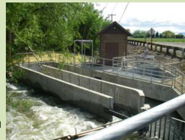
Barnes Road Diversion Fish Screen and Passage Facility
