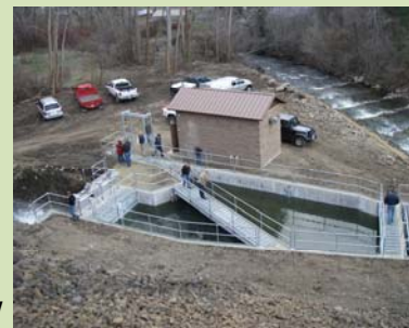
MWDA/Consolidated Fish Screen Facility & Rock Weirs
